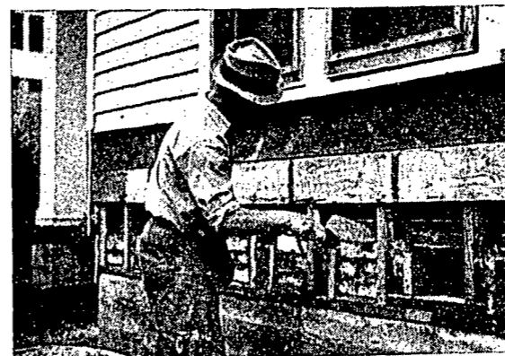
● Mason Laying Fire Stop
